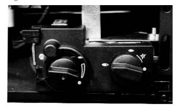
The remote control unit allows operation of the main burner between maximum and pilot only setting. It does not turn the pilot on or off.
