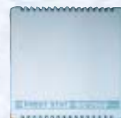
Frost Stat set to 5°C (inside control panel)
