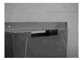
j) Position the fire carefully on the (protected) surface of the hearth and reach into the fire opening. Thread each of the cables vertically downwards through the pair of fixing eyes on the same side of the fire. Thread the free end of the cables through the corresponding circular hole on each side of the lower rear of the fire. Carefully slide the firebox back into the fire opening and pull both cables tight.
