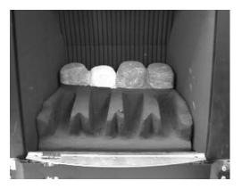
b) Position front ceramic rail on burner front ceramic support and ensure that the locating channel in the front ceramic rail is correctly located onto the lip on the burner front ceramic support. (See fig. 14 below)
