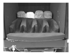
c) Pick pebbles A to E and arrange along the the front rail, ensuring that they are evenly spaced. Use the recess's in the front ceramic rail as a guide for placement. (See fig. 15 below)
