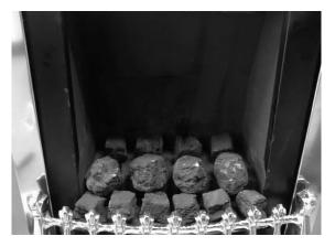
f) Select three of the medium sized coals and arrange along the fuelbed behind the second row of large coals, as shown below in Fig. 18
