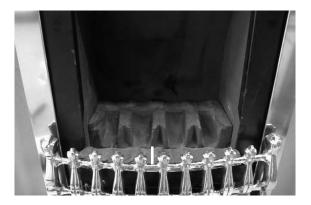
Fit six of the medium sized coals onto the front ceramic rail, ensuring that they are evenly spaced. Use the recess's in the front ceramic rail as a guide for placement. (See fig. 15 below)
