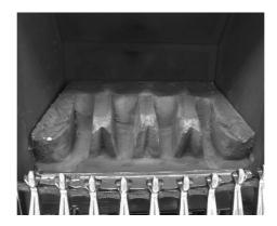
b) Position the two halves of the front ceramic (L/H & R/H) on the locating channel in the front ceramic, ensuring it is located onto the lip on the burner front ceramic support. (See fig. 14 below)
