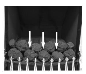
e) Select five of the large coals and arrange along the rear of the fuelbed, using the ribs in the rear of the fuelbed as a guide for placement. (See fig. 17 below)
