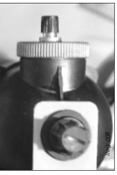
Bleed each radia tor until a continuous jet of water is obtained.
