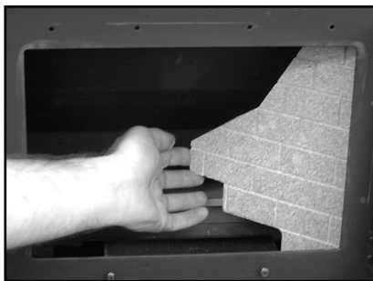
Fig. 3b Fitting the R/H side lining
