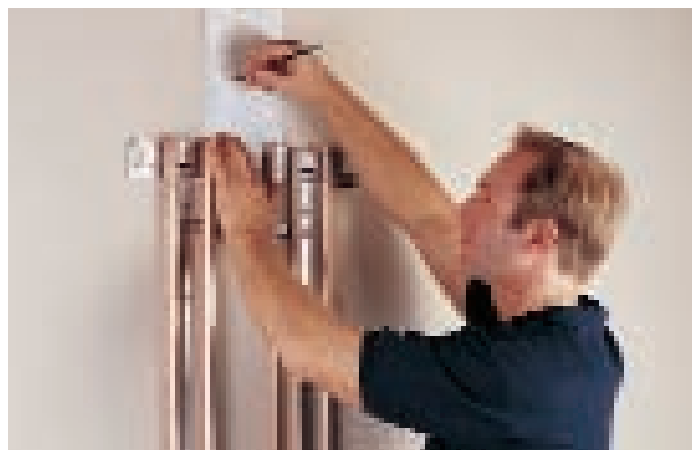
Pre-fixing jig with built-in filling loop
