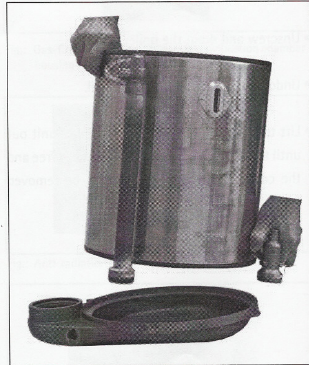
Fig.: Combustion chamber unit / condensate sump
